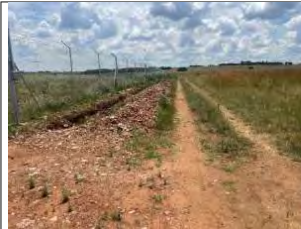
Photo 6: Perimeter fence (left) and access routes (right) along the fenceline.
