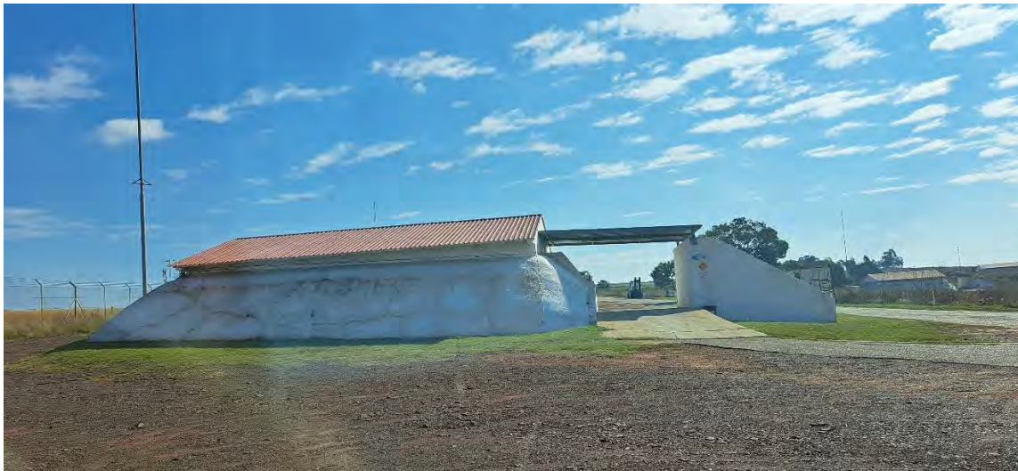
Figure 3-1: Existing magazine storage facilities – Ekandustria
