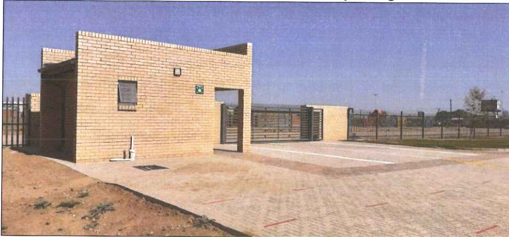
Image 3: Multi-purpose Centre main entrance and parking area
